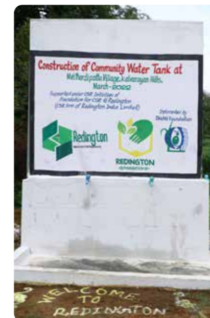
Through Constructing 4 rain water harvesting structures we established water storage tank with a capacity of storing - 52 Kilo Litres
