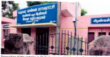
Renovation of the complex in Thalakuppam, which has six toilets each for men and women, was completed three months ago | P RAVIKUMAR
