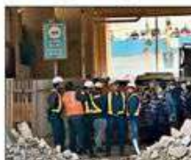
DMRC has begun a review on the incident at Gokulpuri metro station.
