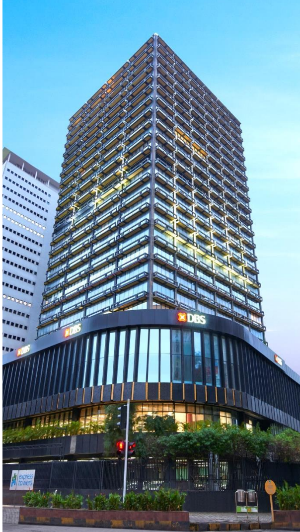
Express Towers Mumbai (0.5 msf)
