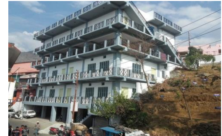
Construction of Commercial cum parking complex at Gopeshwar
