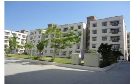
Construction of Residential project at Haridwar
