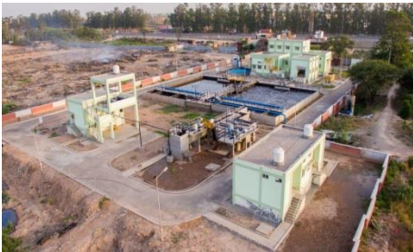
Water supply and sewerage project in Rajpura Punjab
