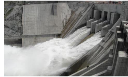
450 MW Baghlihar Hydro Electric Power Project, Chanderkot, District Ramban
