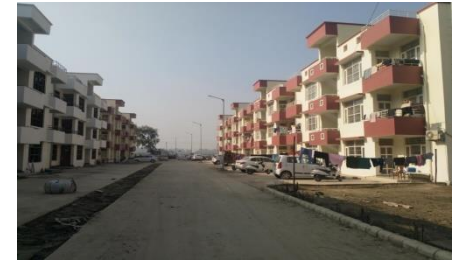
Construction of Police staff quarters at Madhuban
