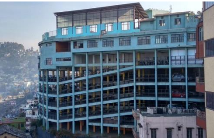
Construction of Commercial cum parking complex at Almora
