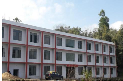
Construction/ Infrastructure Development of Kohima College, Kohima, Nagaland
