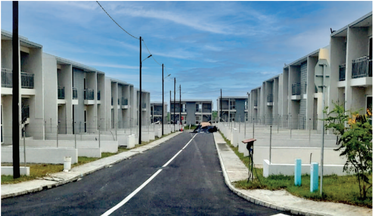
Social Housing Project at Mare Tabac Site, Mauritius
