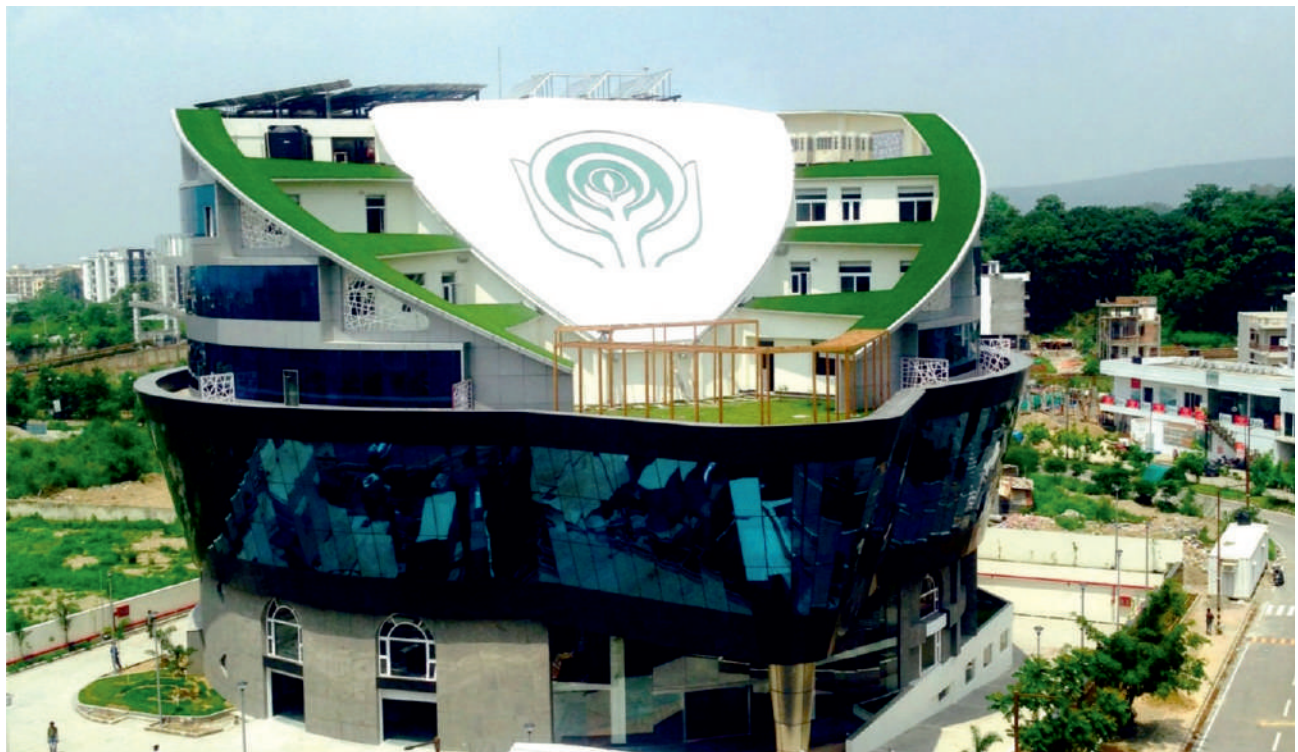
NABARD Regional Office Building, Dehradun, Uttarakhand
