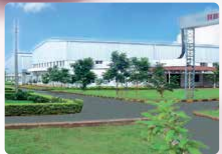
NANDIGAON Near Hyderabad, Telangana Product line: PLT, Lithium-Ion and Submarine Batteries
