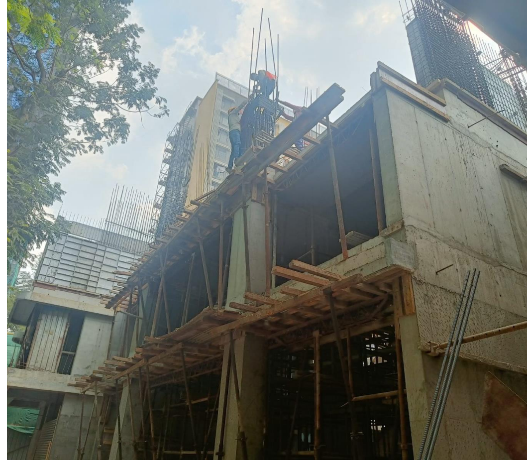
2nd Floor Slab Casted
