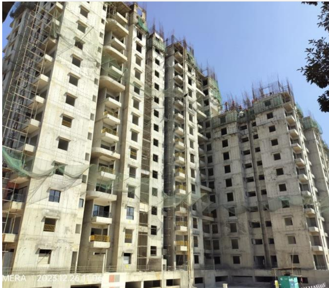
Tower AB - South View
