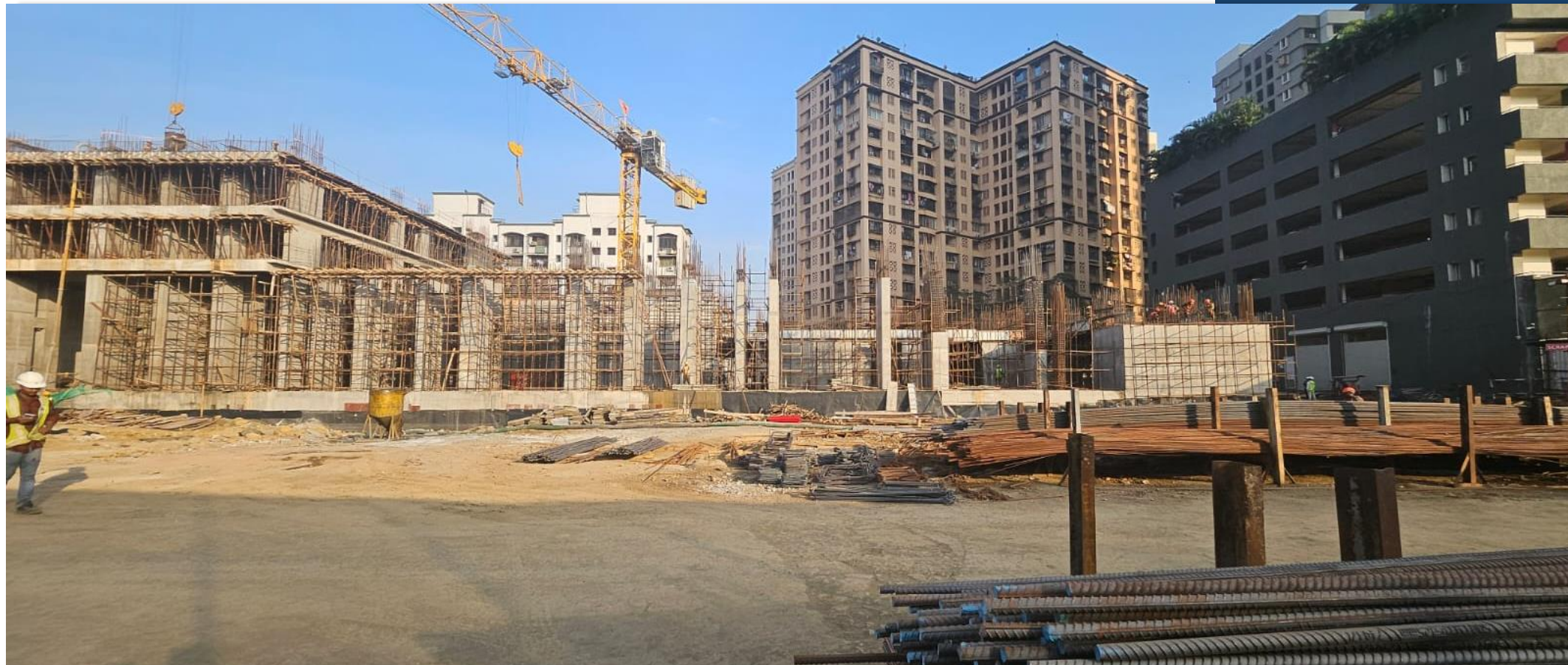
Tower B – Podium WIP
