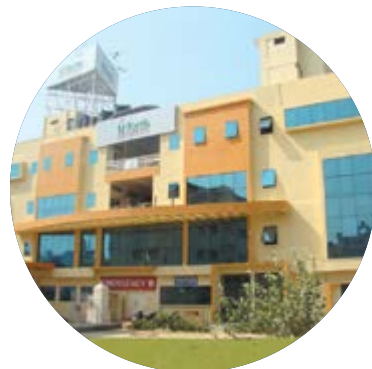
Fortis Hospital, Nagarbhavi, Bengaluru
