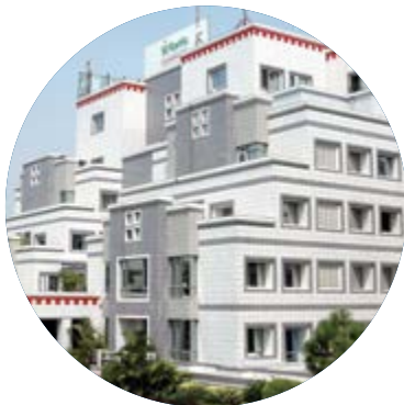
Fortis Ft. Lt. Rajan Dhall Hospital, Vasant Kunj, New Delhi
