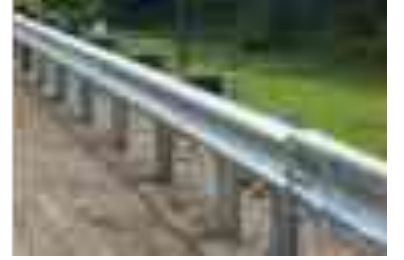
Metal Beam Crash Barrier
