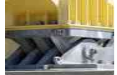
Bearing & Expansion Joint
