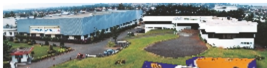
Menon Bearings plant at Kolhapur,
