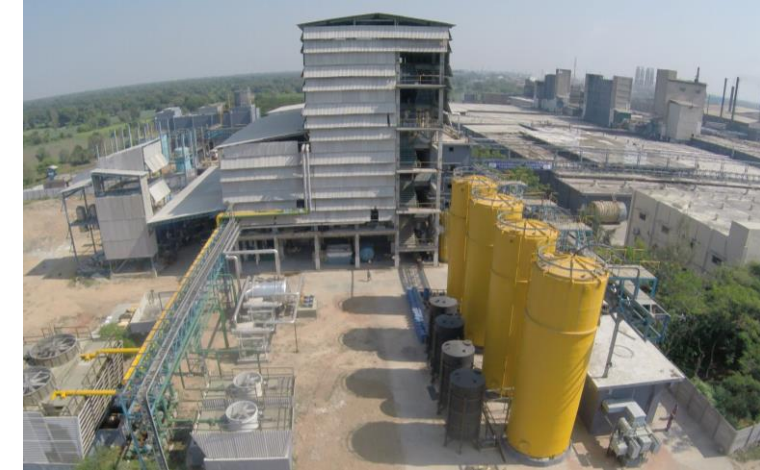
Multiple Effect Evaporator Plant (MEEP)
