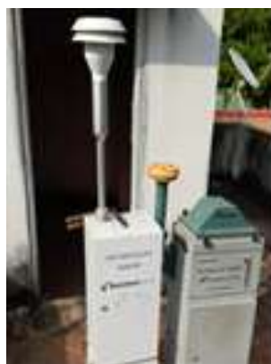
AAQ Station installed in Mudhanai, Neyveli
