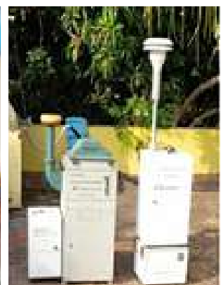
AAQ Station installed in Umangalam, Neyveli
