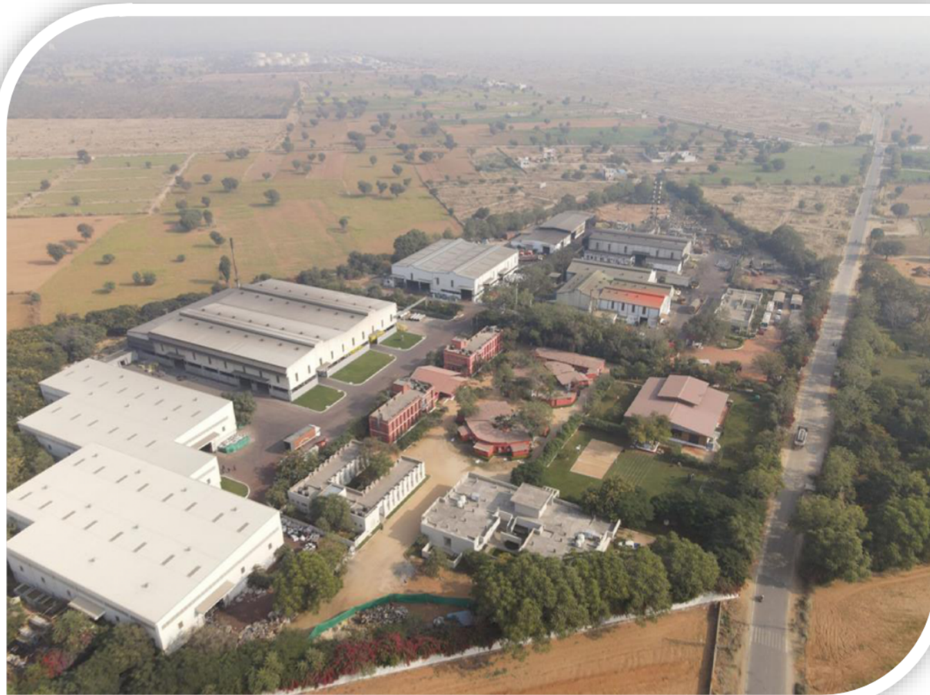
Phagi Plant's Full Ariel View
