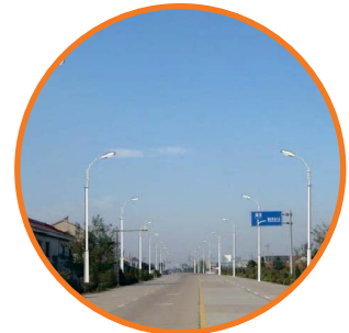
Dakshinanchal Vidyut Vitran Nigam Limited Project-Village & Highway Electrification Products Used- Steel Tubular Poles
