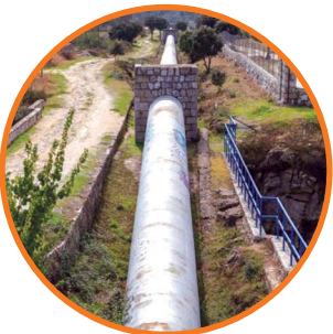
UP & Utrakhand Peyjal Nigam Project-Water distribution Products Used-GI Pipes
