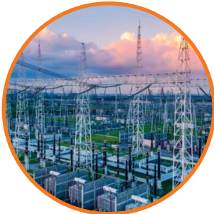
Madhyanchal Vidyut Vitran Nigam Limited Project-Village & Highway Electrification Products Used- Steel Tubular Poles
