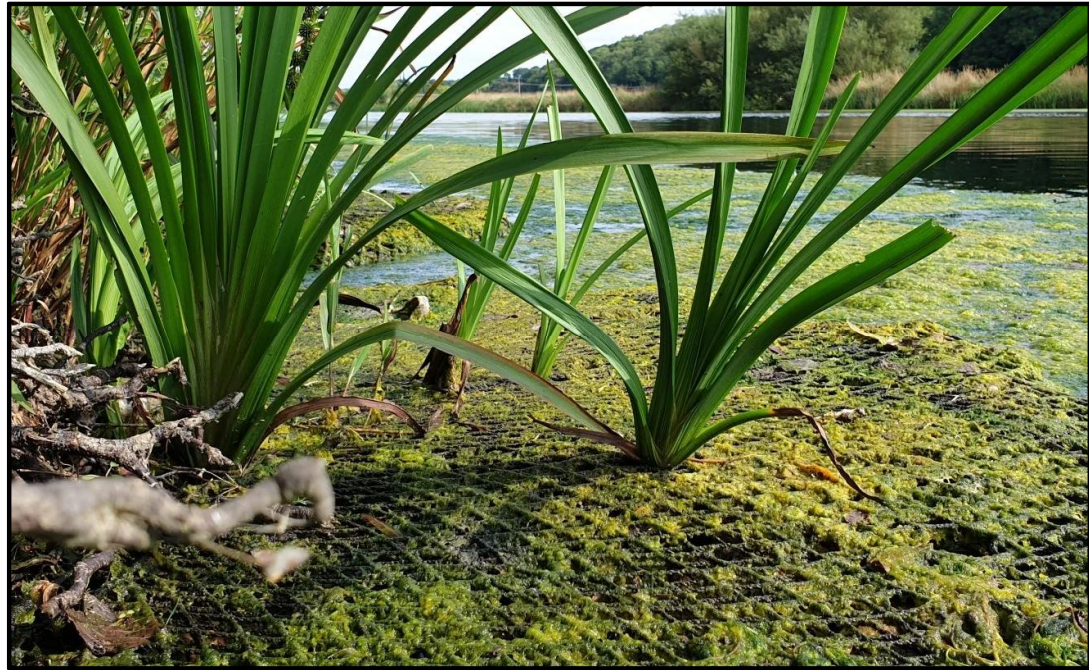
Erosion Control and Scour Protection along a river bank in Cumbria, North England
