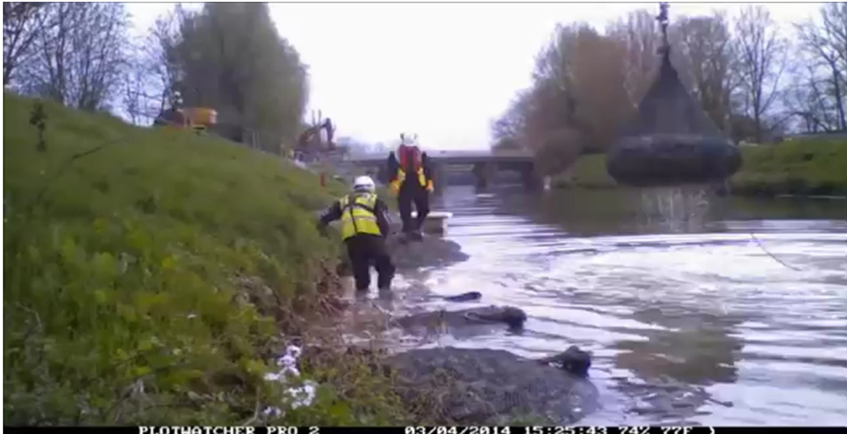
Installation of Erosion Control and Scour Protection AquaRockBag in England
