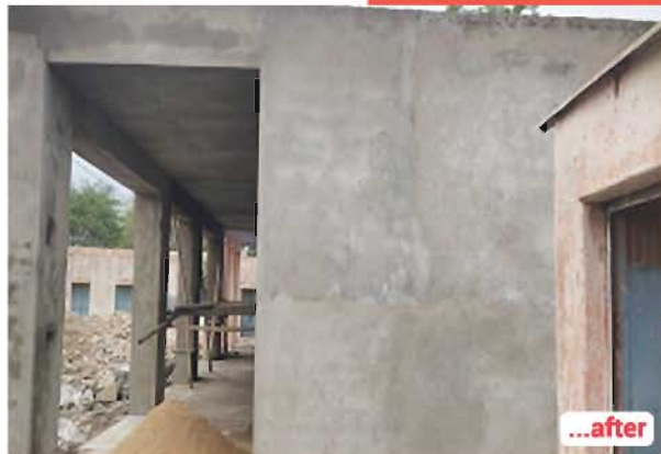
Renovation work near completion
