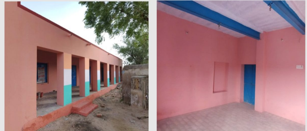
Kanpur School repair work
