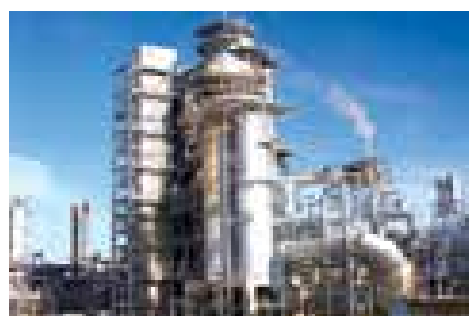
HPCL Bhatinda & Manglore Refinery Project Project: Refinery Project Products Used: Pipes
