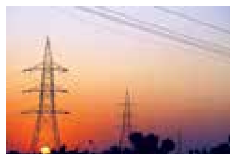
Power Projects Project: J&K Rural electrification Products Used: Steel Pipes & Poles
