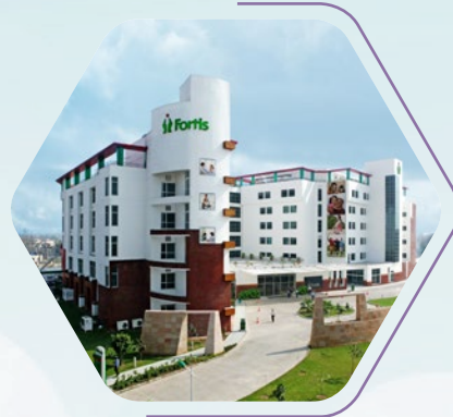
Fortis Hospital Shalimar Bagh, New Delhi
