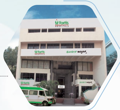
Fortis Hospital, C.G. Road Bengaluru
