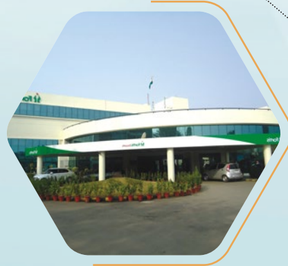
Fortis Escorts Hospital Faridabad
