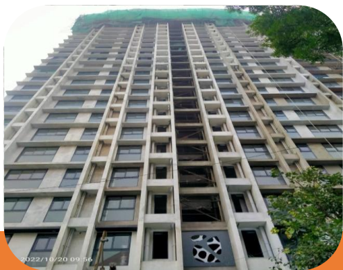
Super Structure completed in Feb 2022
