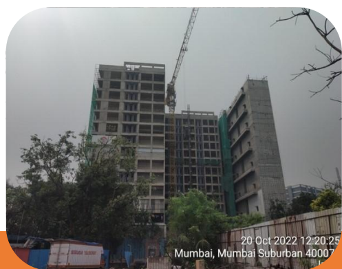
RCC work completed
