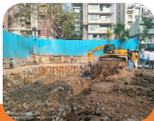
Piling work completed
