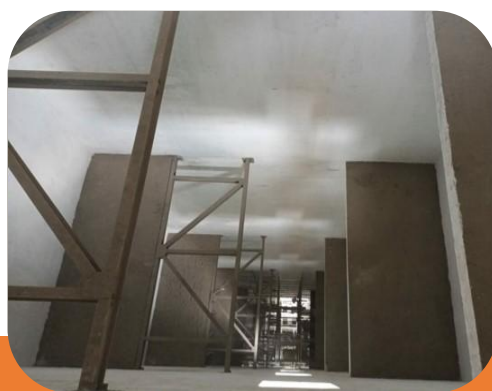
MEP & Finishing - WIP
