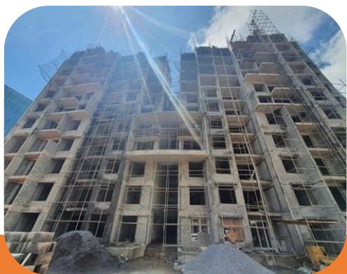
Nucleus C Under Construction
