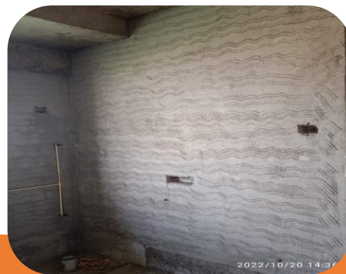
MEP & Finishing - WIP
