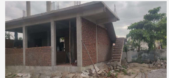
Construction of Mahila Bhavan at Sangareddy District of Telangana
