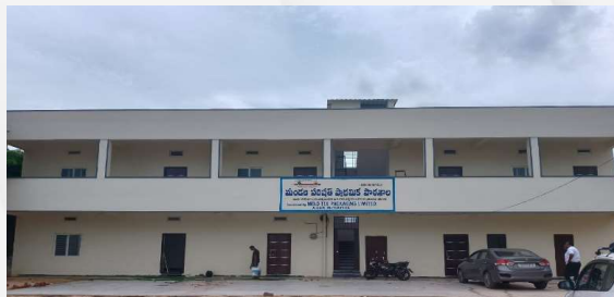
Construction of School Building at Annaram, Medak Dist. of Telangana
