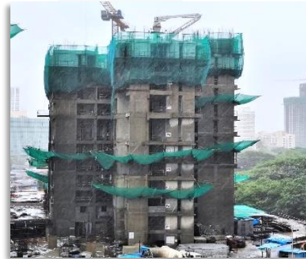
Tower (B) 3 rd Floor Slab Completed
