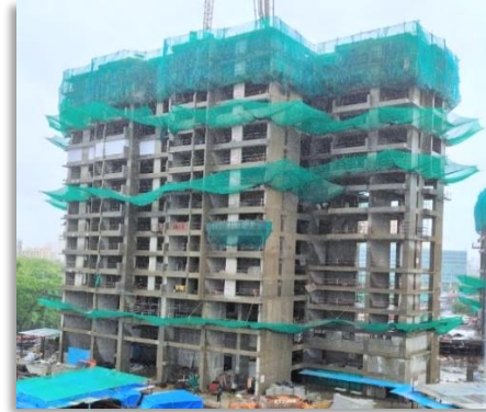
Tower (A) 7 th Floor Slab Completed
