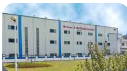
Paints Plant, Dadra
