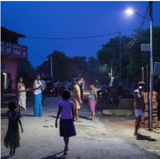
Village Development - Construction of Toilets and Erection of Street Lights Enhancing rural infrastructure in Mattapalli, Telangana, by constructing toilets and erecting street lights.
