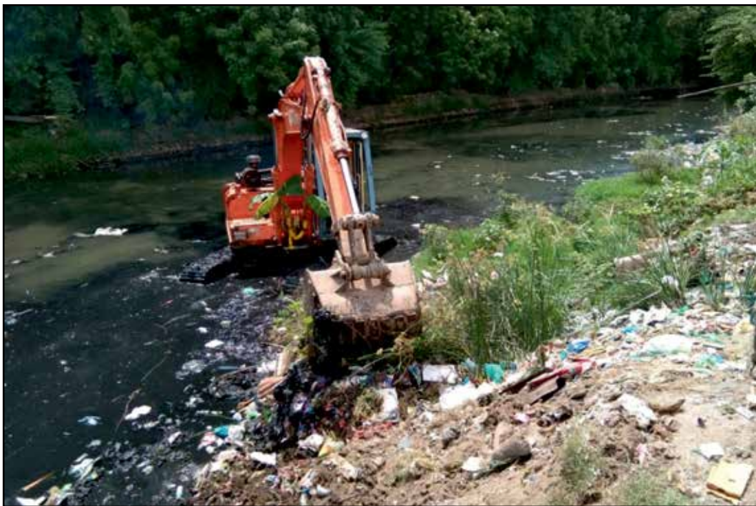
Desilting of Water Bodies - Uppanar Canal
