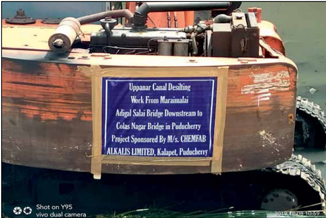
Desilting of Water Bodies - Uppanar Canal
