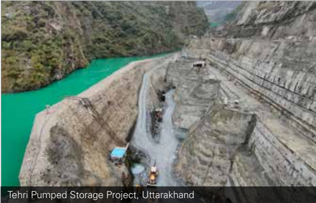
Tehri Pumped Storage Project, Uttarakhand
