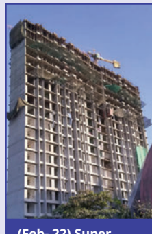
(Feb- 22) Super Structure Completed
