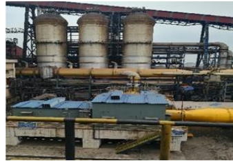
BLAST FURNACE, STEEL PLANT WORK, JSPL, ANGUL
