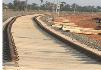
GDV-MTM 37 ,DOUBLING & ELECTRIFICATION WORKS , RVNL
