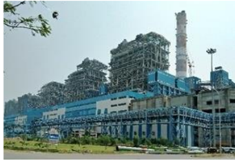
3X660 MW STPP, BOILER & CRITICAL PIPING, U#1,2&3, BARH, DOOSAN
