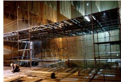
CUPLOCK SCAFFOLDING ERECTION 800MW,MUNDRA
