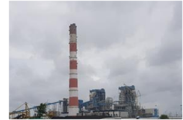
2X660 MW STPP, BOILER, ESP U#1&2, SOLAPUR, BGRESL
