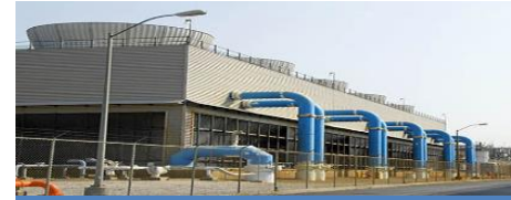
Infrastructure Construction (Civil)
