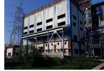
1X500MW, FGUTTP, CIVIL, STRUCTURAL AND ARCHITECTURAL WORK FOR BTP, BOP & CHP, UNCHAHAH, NBPL
