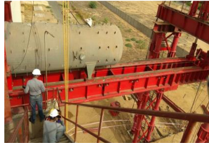
HP HEATER REPLACEMENT 800MW ,CGPL MUNDRA2
