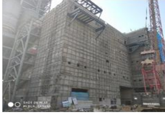
1X800 MW TPSS, CIVIL, STRUCTURAL AND ARCHITECTURAL WORK UNIT-12, KOTHAGUDEM, BHEL
