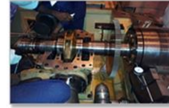
228MW, STEAMTURBINE,SABIYA, KUWAIT, MAIN OIL PUMP OVERHAULING
