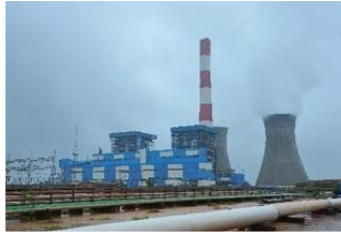
2X600MW TPP, BOILER & STG, MANGALORE, LANCO (COMPLETED)
