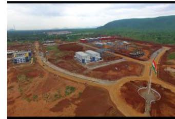
INFRASTRUCTURE DEVELOPMENT WORK, AP MEDI TECH ZONE, VIZAG
