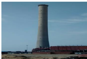
1X500 MW, FGUTTP, CIVIL, STRUCTURAL AND BOP & CHP, UNCHAHAH, NBPL
