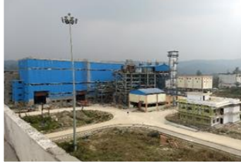
1X100 MW CCPP, BALANCE CIVIL & STRUCTURAL WORKS, NAMRUP, BHEL (COMPLETED)
