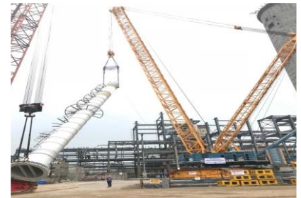
UREA REACTOR TANK INSTALLATION AT RAMAGAUNDAM, TELANGANA
