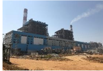
2X660 MW IBTPS, STRUCTURE & STG, BANHARPALLI, BHEL
