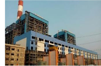
2X800 MW, YTPS, CIVIL, STRUCTURAL AND ARCHITECTURAL WORKS RAICHUR, BHEL (COMPLETED)
