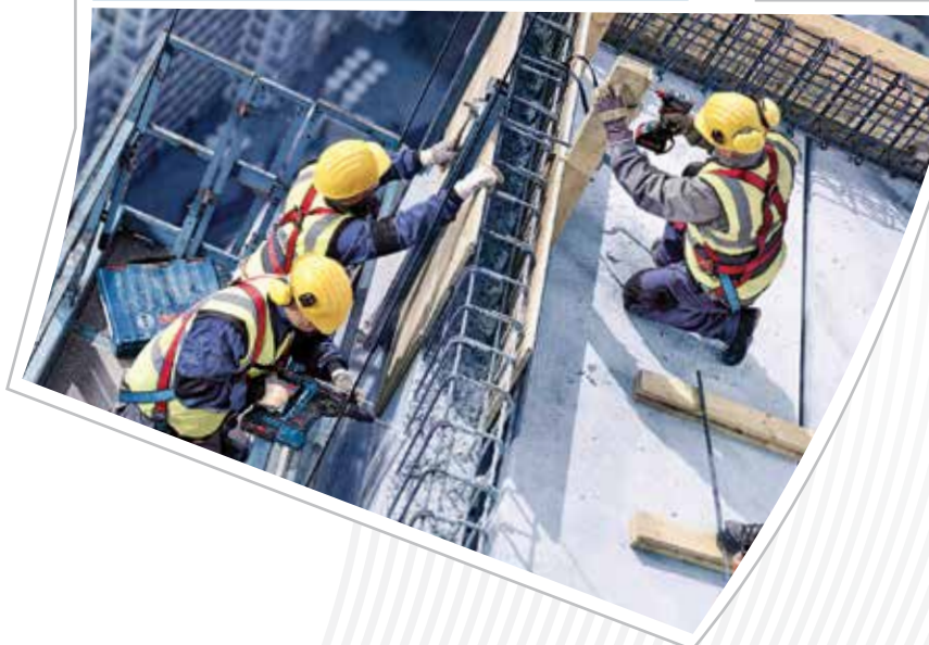
Workers using a Bosch's Cordless Power Tools
