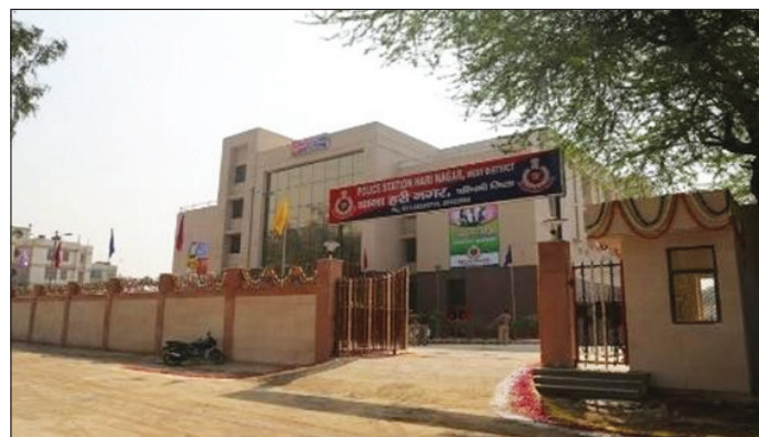
Construction of Police station & Residential Quarters, Hari Nagar, Delhi for MHA, Delhi Police through RITES Ltd.
