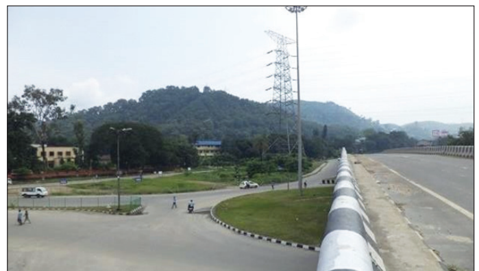
Widening & Strengthening of existing National Highway from 2 lane to 4 lane of Sonapur to Guwahati section of NH-115 (earlier NH 37) for NHAI.
