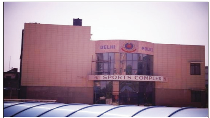
Police Station & Residential Quarters at Kondli, New Delhi for MHA, Delhi Police through RITES Ltd.
