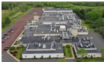
CDMO: Acquired solid oral dosage facility in Sellersville, Pennsylvania
