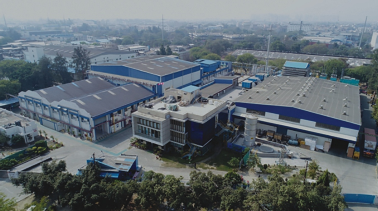
Noida Plant- Manufacturing facility for Liquid inks, News colour inks
