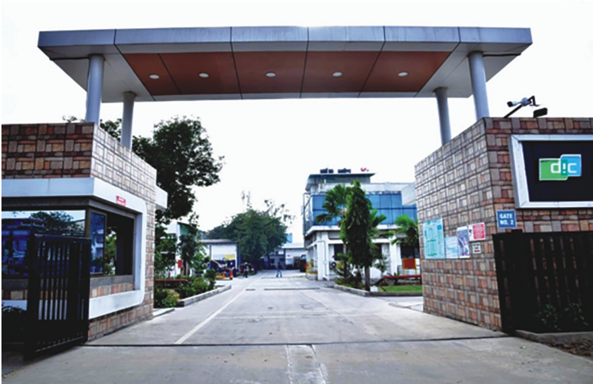
Ahmedabad Plant- Manufacturing facility for News Black inks, Offset aquatic inks
