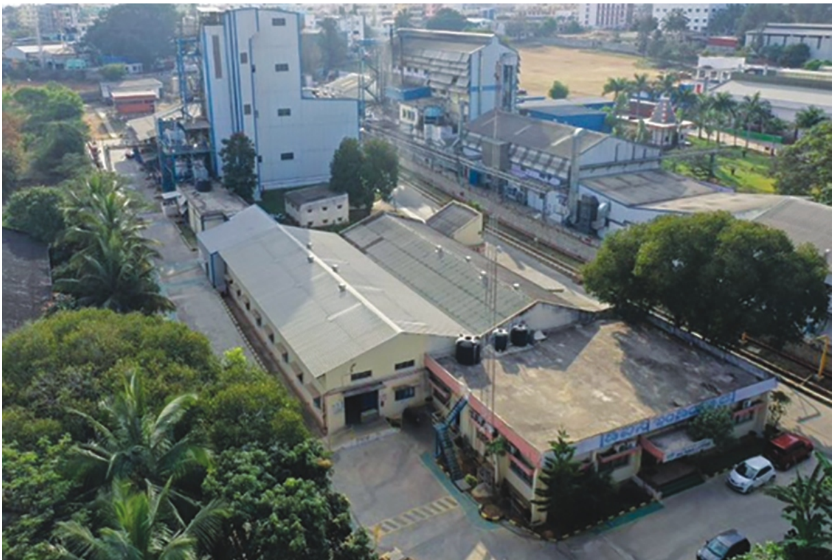
Bengaluru Plant - Manufacturing facility for Adhesives and PU Resins
