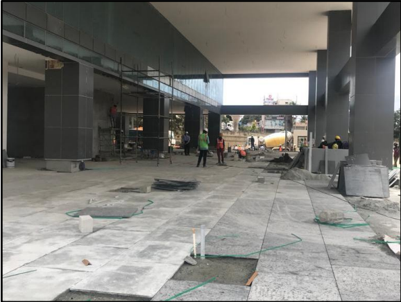
Internal View of the Subject Property
