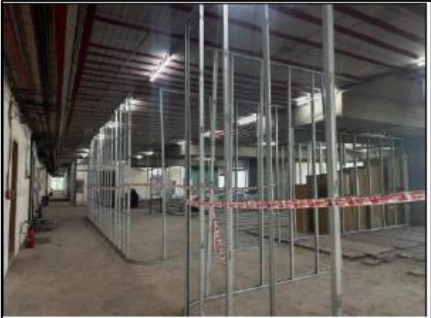
Internal View of the Subject Property
