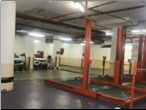
View of the Basement Car Parking
