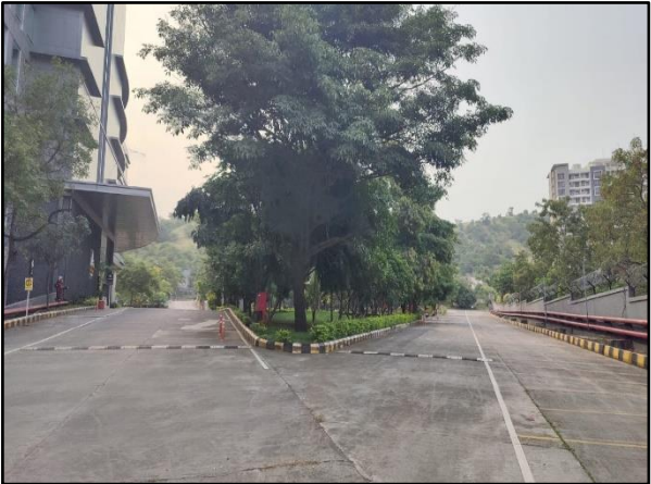
View of the Internal Access Road
