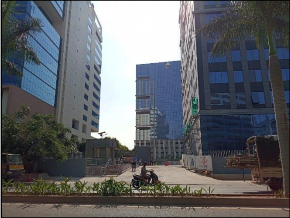
External View of the Subject Property
