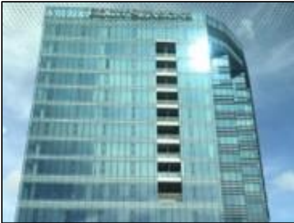
External View of the Subject Property
