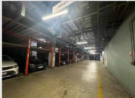
View of basement car parking
