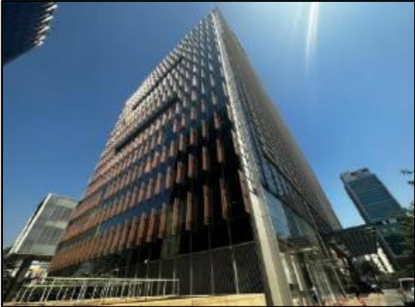
External View of the Subject Property
