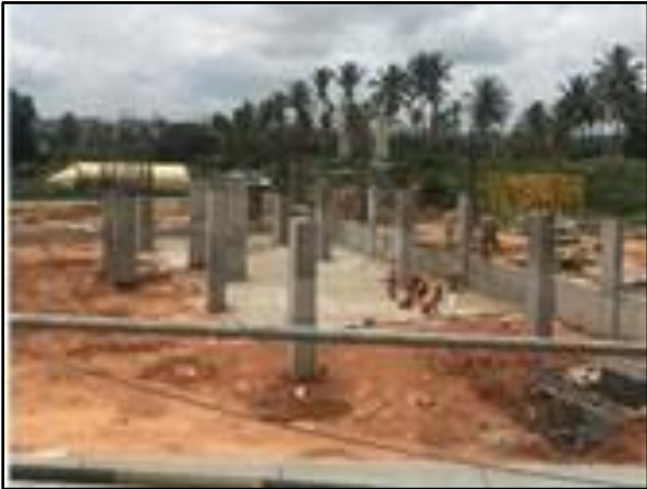
View of the Construction Progress
