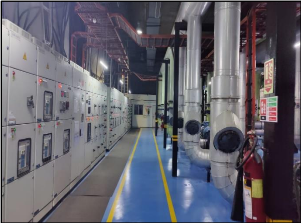
Internal View of the Subject Property
