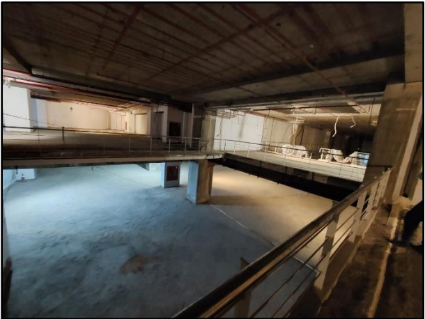
View of the Internal Vacant Space
