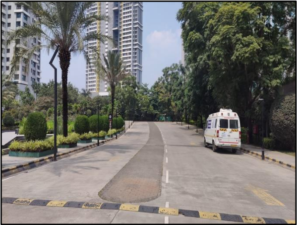
View of the Internal Access Road
