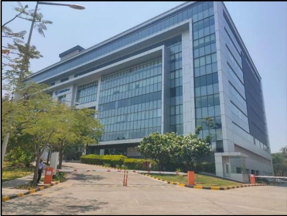
External View of the Subject Property
