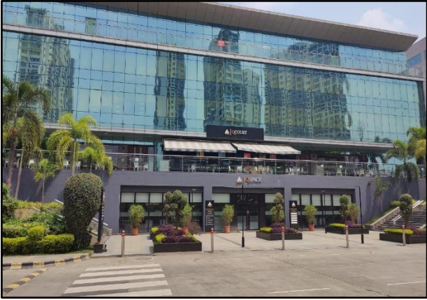
External View of the Subject Property
