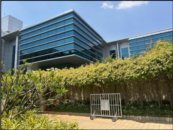
External View of the Subject Property
