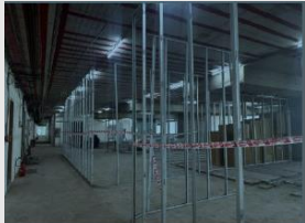
Internal view of Subject Property
