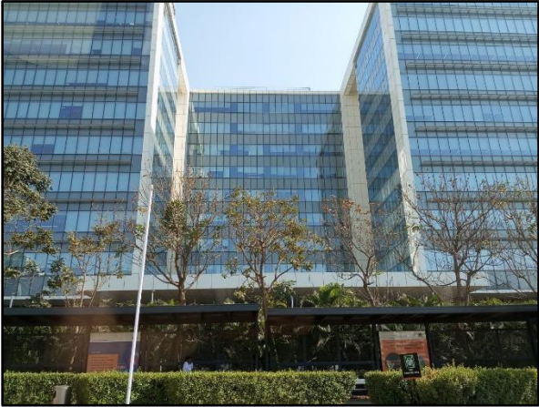
External View of the Subject Property
