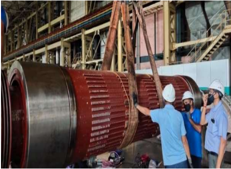
Successful repair 210MW BHEL Gen. rotor at Khaperkheda
