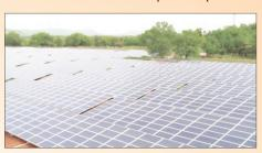
partly for KIOCL units at Mangalore, your Company had commissioned 5.0 MWac (6.5 MWp) Solar Power Plant at Kathrikehal Village, Chikkanayakanahalli, Tumkur District in Karnataka. The installation of plant was successfully completed with project cost of ₹24.44 Crores (Excluding GST). The estimated power generation from the plant is 10 million Kwh per annum (10,000 M Watt hour).
