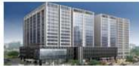
HQ and R&D center
