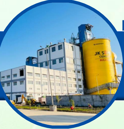
Hamirpur Grinding unit Capacity 2MTPA
