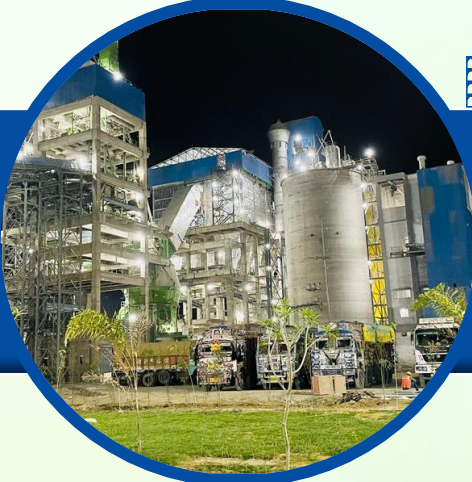
Panna Integrated unit Capacity 2MTPA
