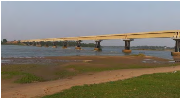
Bridge no. 134 over River Mahanadi
