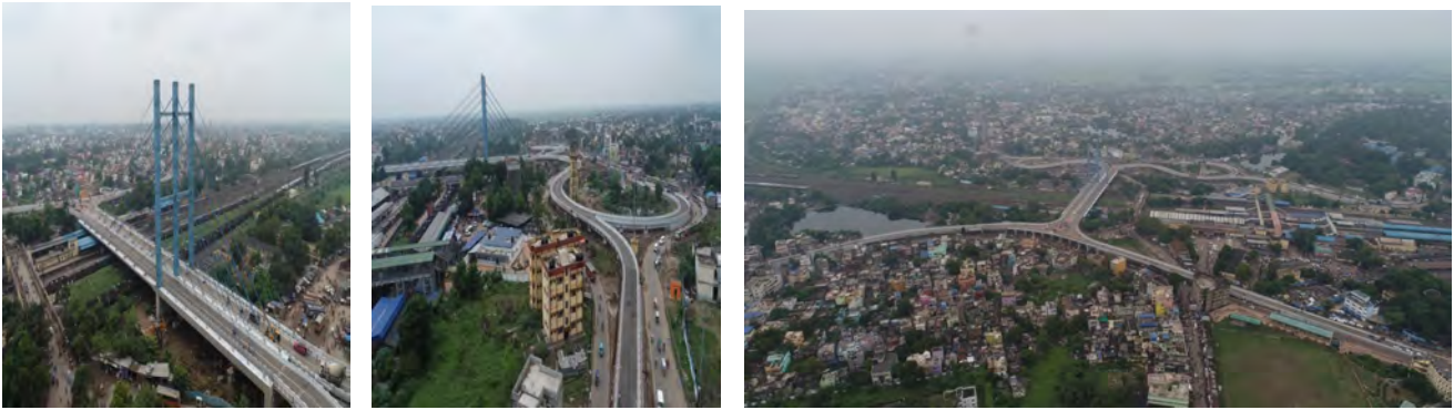
4-lane Cable Stayed Bridge over busy Barddhaman Yard along with its 3.5 Kms long approaches commissioned in Sep 2019.
