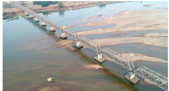
Bridge no. 12 on river Brahmani
