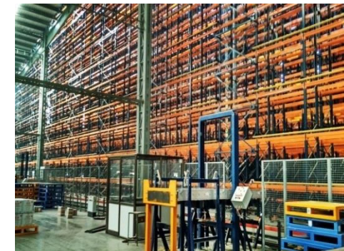
Automated Storage and Retrieval System
