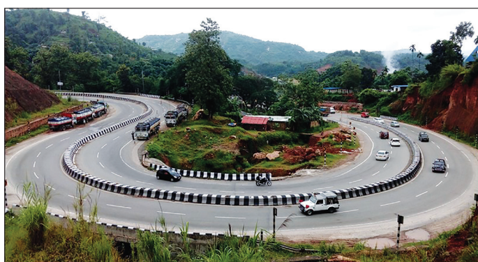
Widening & Strengthening of existing National Highway from 2 lane to 4 lane of Sonapur to Guwahati section of NH-115 (earlier NH 37).
