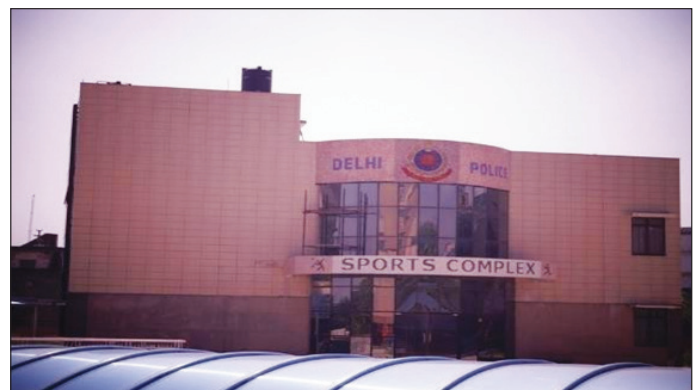
Police Station & Residential Quarters at Kondli, New Delhi for MHA, Delhi Police through RITES Ltd.
