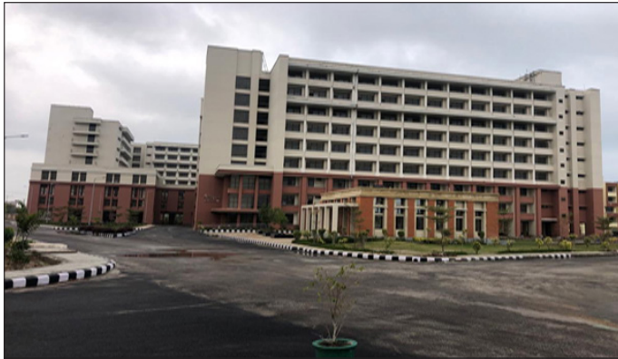
Construction of National Law University, Rai in Sonapat District, Haryana for PWD (B & R), Haryana
