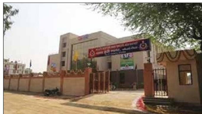
Construction of Police station & Residential Quarters, Hari Nagar, Delhi for MHA, Delhi Police through RITES Ltd.
