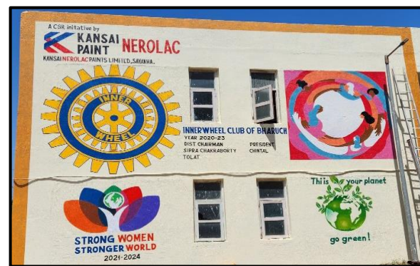
Boundary walls were painted with various environmental slogans at Shri K J Govt. Polytechnic Institute, near Sayakha plant
