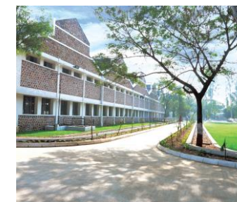
Jain Plastic Park Alwar (Rajasthan) Plastic Piping Plant, Solar and PFS
