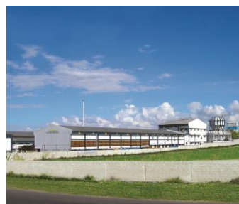
Jain Plastic Park Hyderabad (Telangana) Plastic Piping
