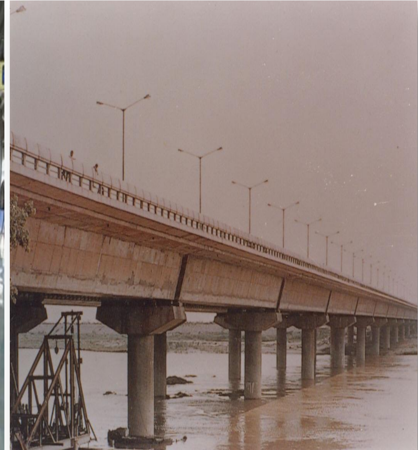
BRIDGE ACROSS RIVER YAMUNA, NEAR ISBT DELHI
