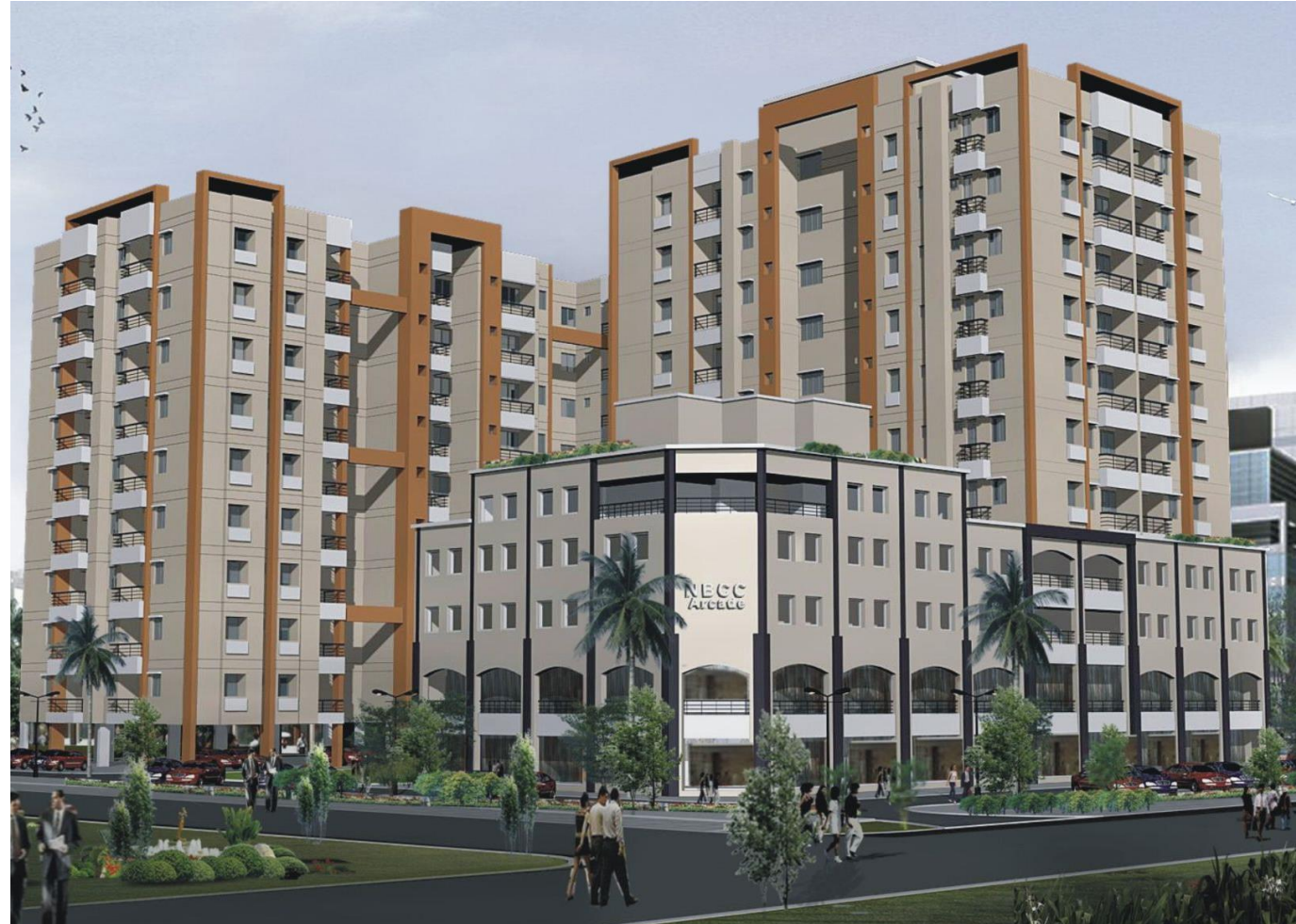
NBCC TOWER, BAHADURPUR, PATNA
