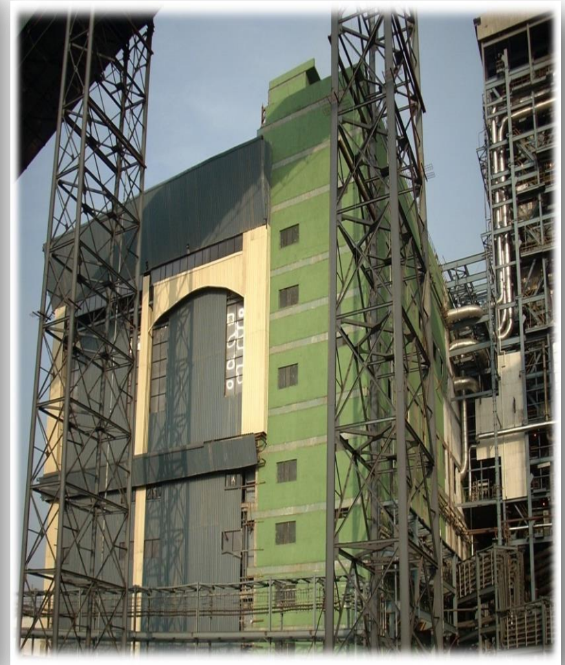
POWER HOUSE - KORBA (CHHATTISGARH)
