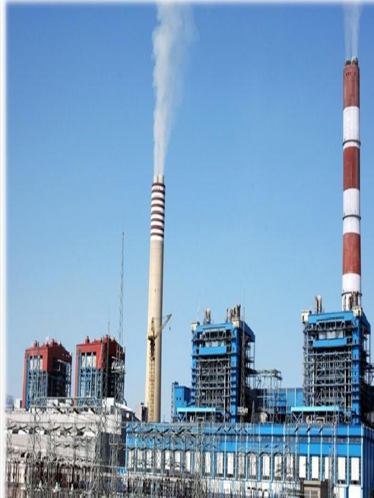
MAIN PLANT, RIHAND (UP)
