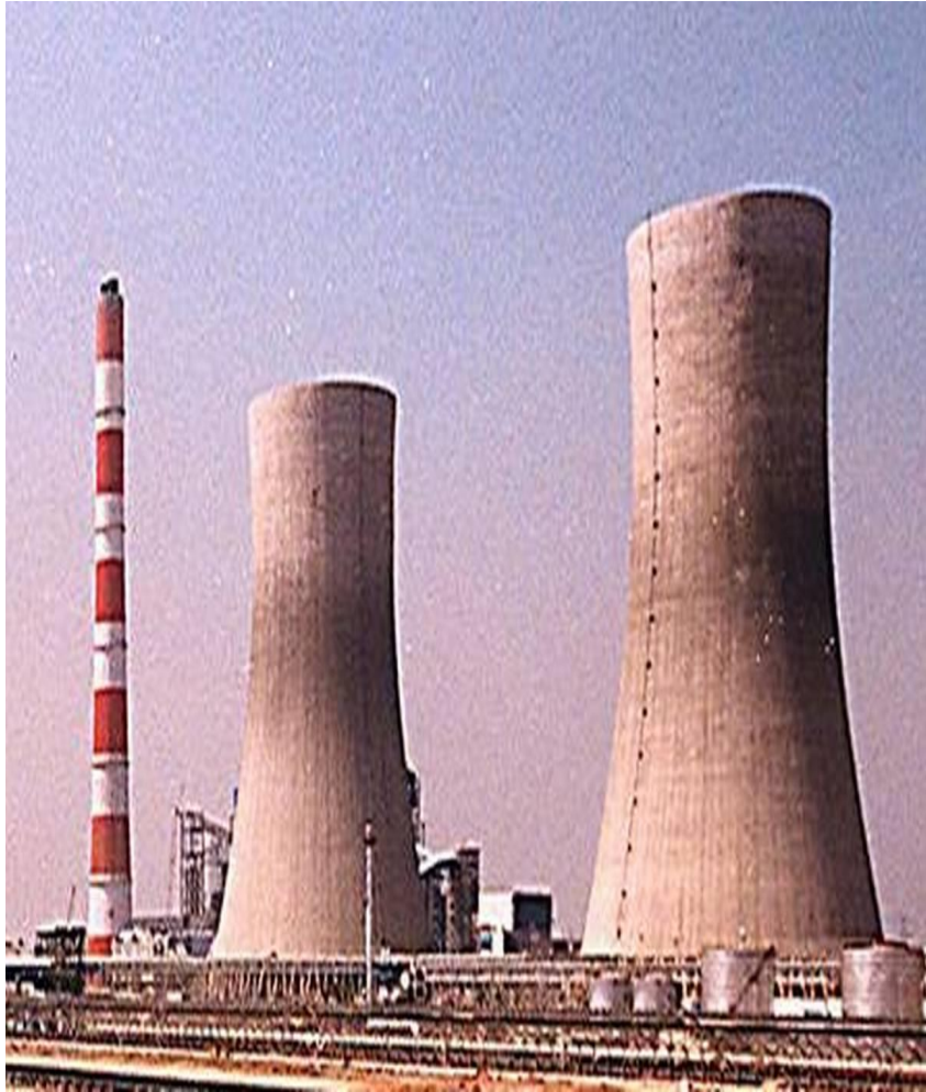
COOLING TOWER & CHIMNEY,(ANDHRA PRADESH)
