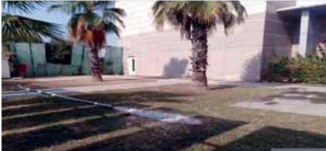
RO water reject reused for landscaping
