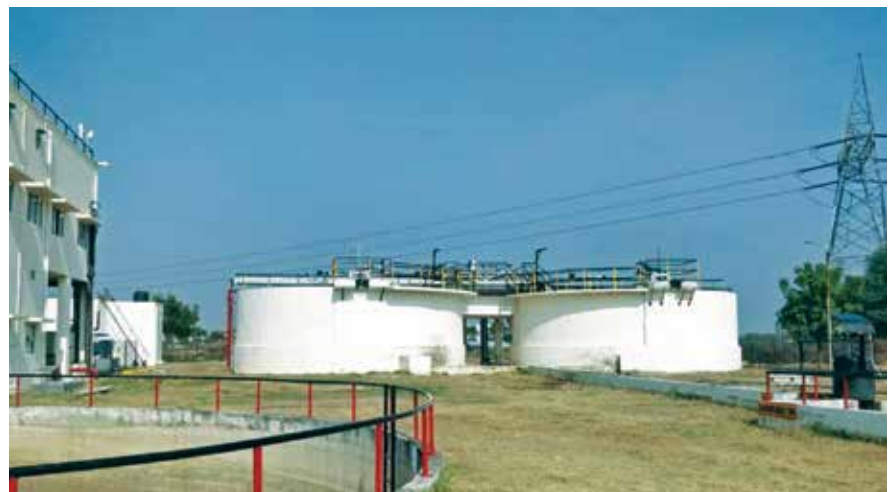
Sewage Treatment Plant at Mahindra World City, Jaipur
