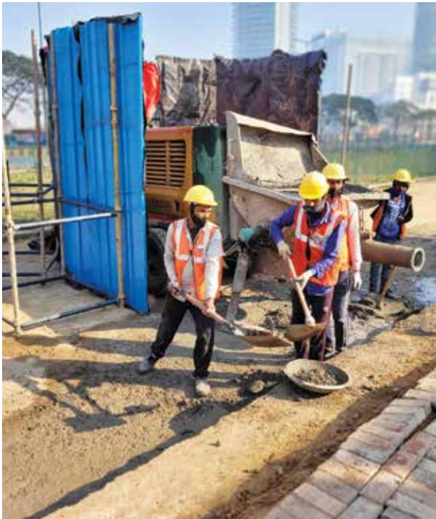
Rockwool insulation around cement mixer for noise pollution mitigation at Mahindra Luminare
