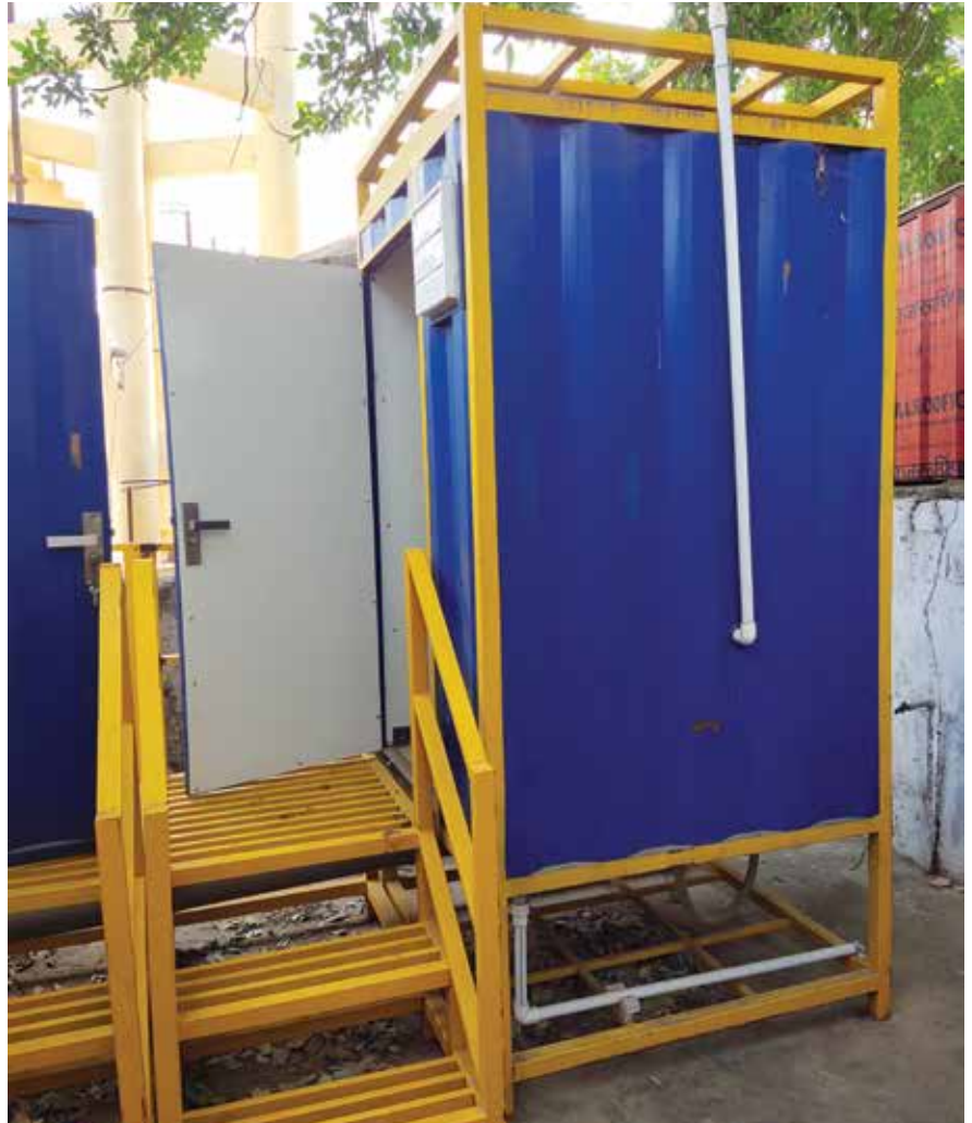
Construction of Bio-Toilets in Government school, near MWC Jaipur
