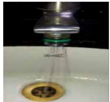
Use of aerators for water taps
