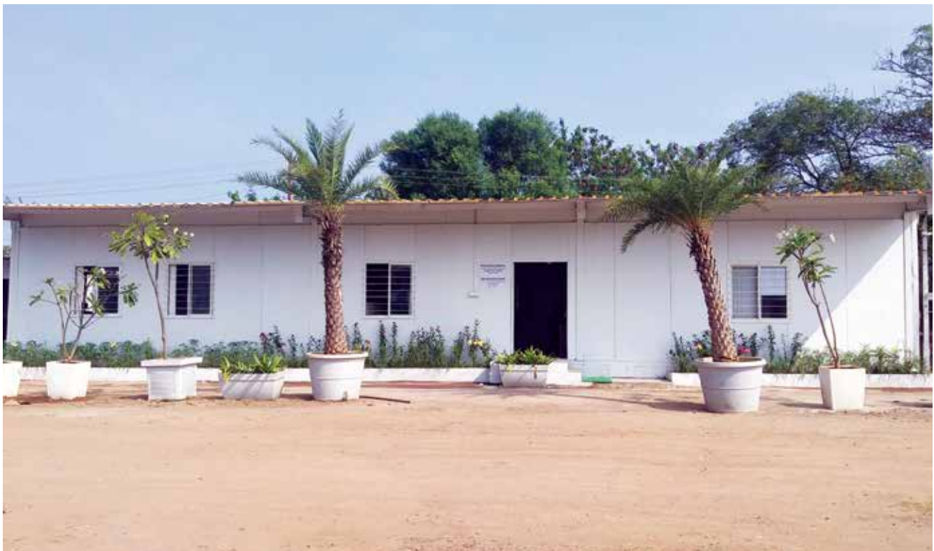
New project office constructed using reusable waste from old office at Mahindra Happinest Tathawade
