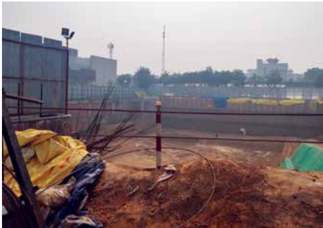
Treated wastewater sprinkling for dust suppression during construction
