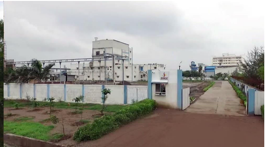
Dahej SEZ Plant
