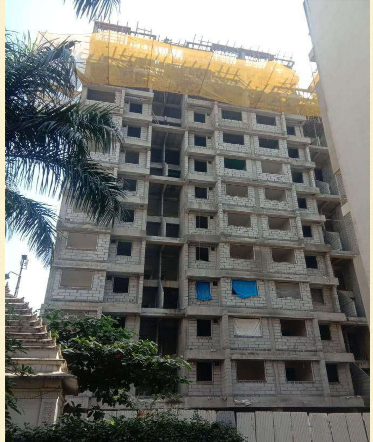
RCC work up to 12 th slab level completed
