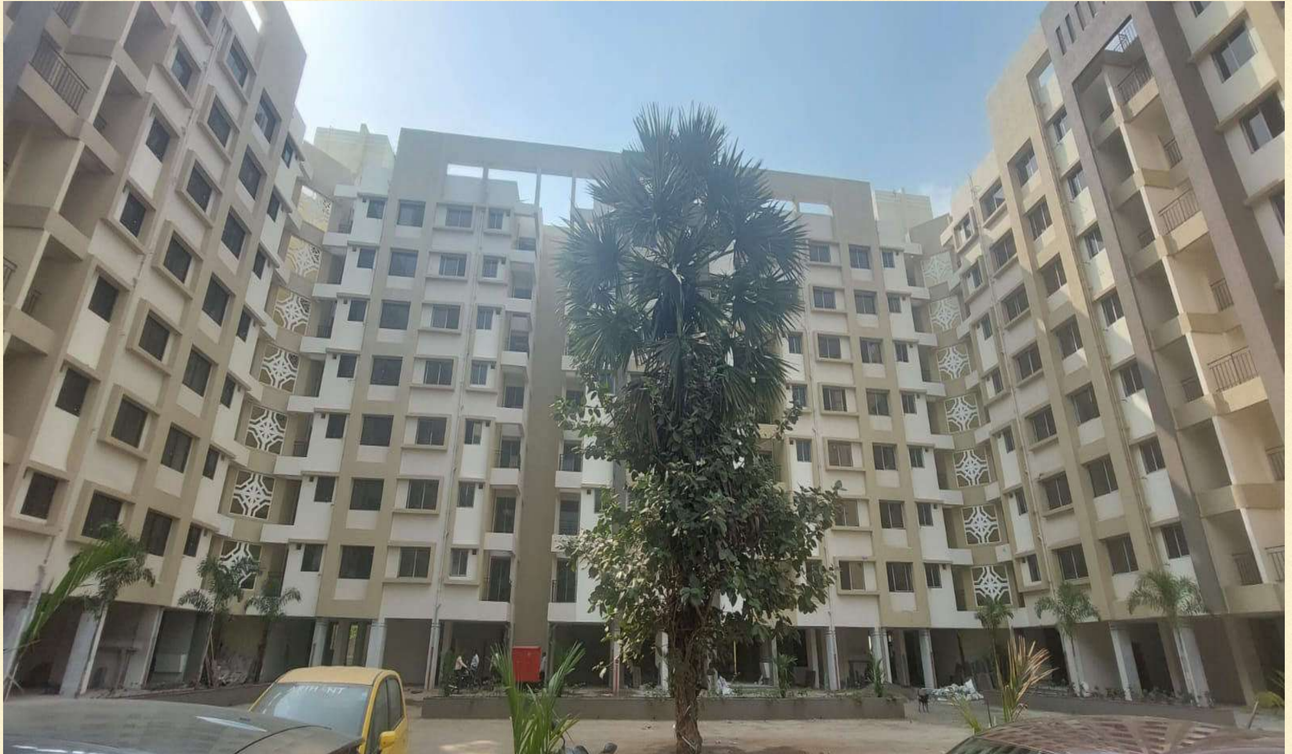
Doors & Windows completed in J, K, L & M wings
