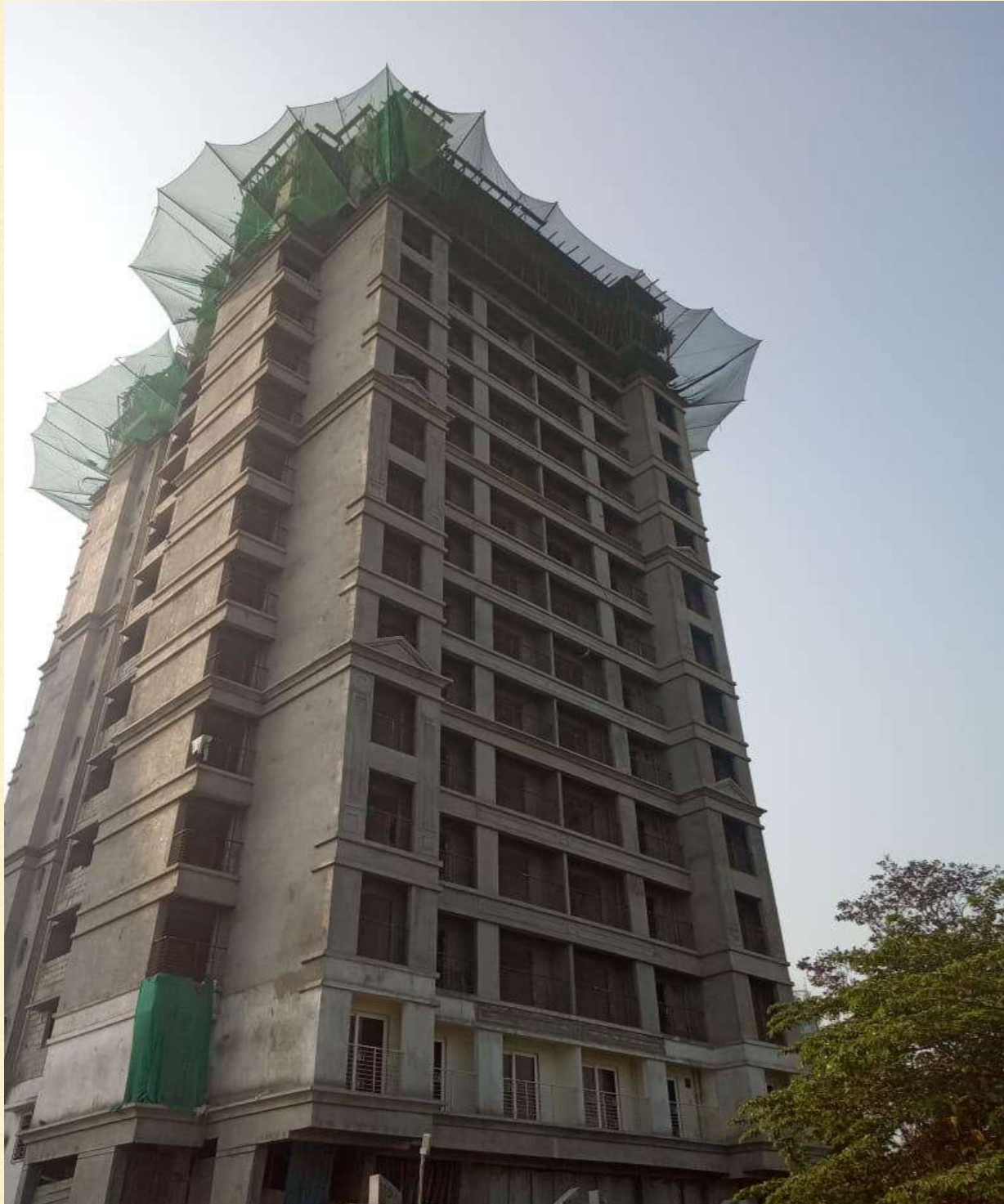
Flooring, tiling, kitchen works in progress
