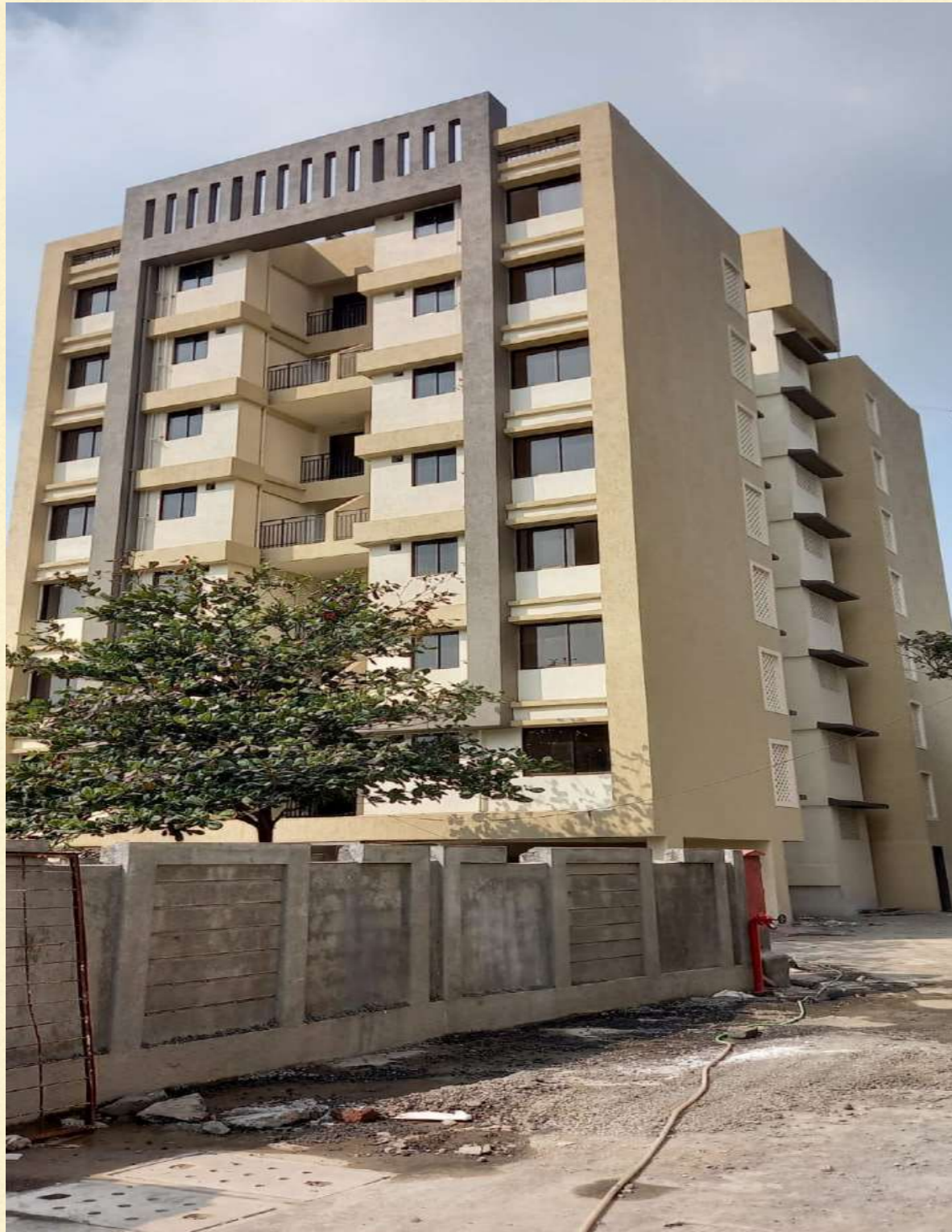
Flooring & Tiling, Doors & Windows completed
