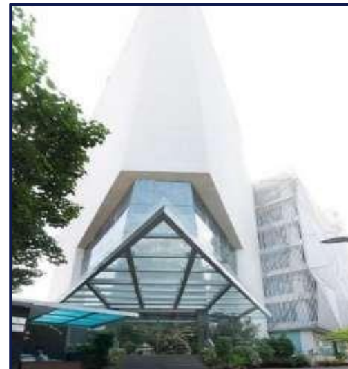
CCIL Bhavan Phase I : Upto 6 th floor
