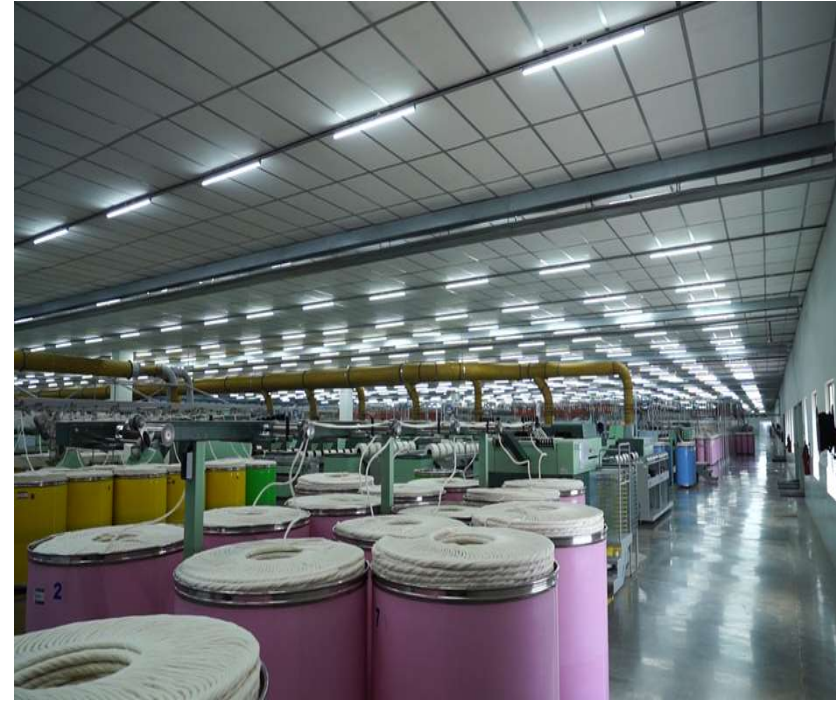
Electrification work of Spinning Mills
