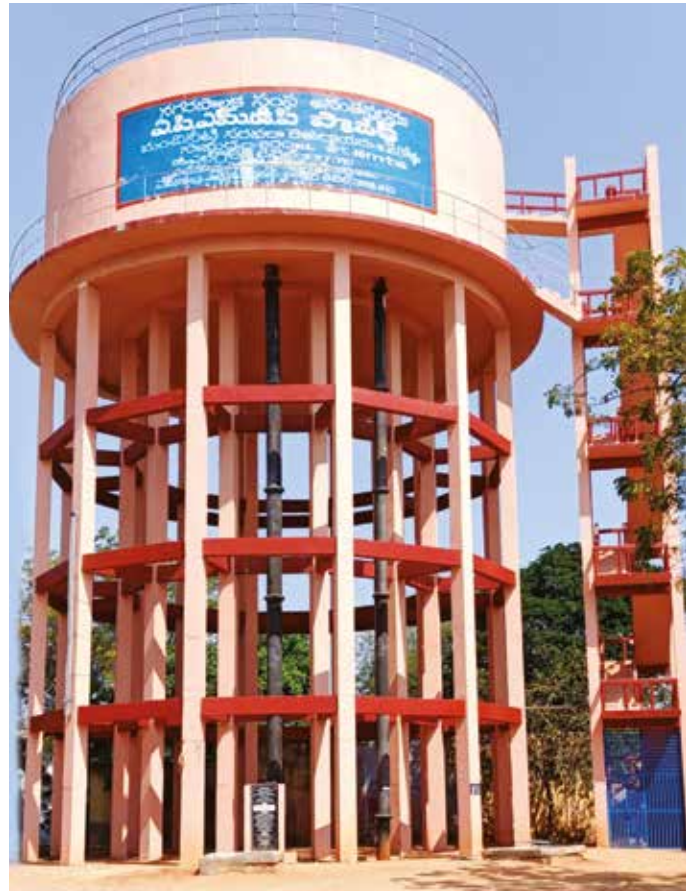
600 KL x 16 Mtr Staging ELSR for Ananthapuramu Comprehensive Water Supply Improvements, in Andhra Pradesh.
