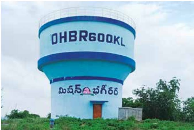
600 KL OHBR at Mallannagutta for Balkonda (TDWSP) Project, in Telangana.
