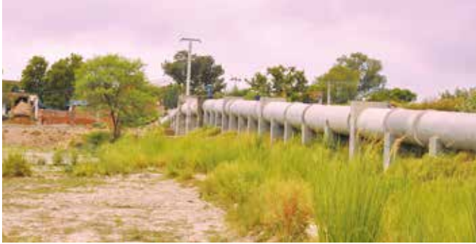
1200 mm dia BWSC pipeline at Santhi Village for Firozabad WSS, in Uttar Pradesh.
